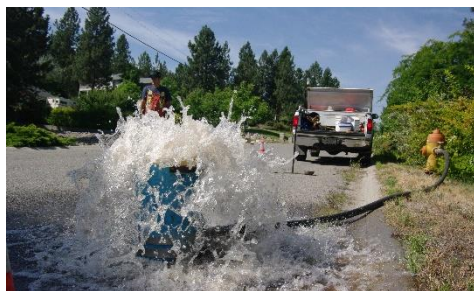
Flushing in Progress
