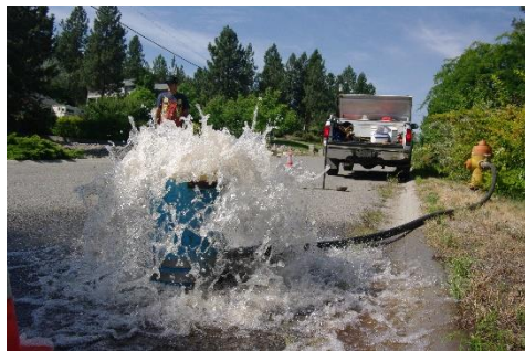
Flushing in Progress
