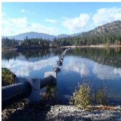
McKinley Bypass pre-sinking
