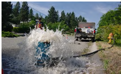
Flushing in Progress
