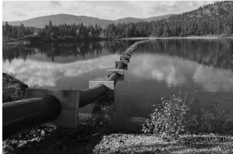
Bypass under Construction at McKinley Reservoir
