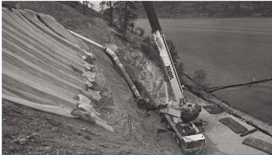
Perfect alignment of 42" pipe by Hayter Construction using 200 ton crane, August 18th.
